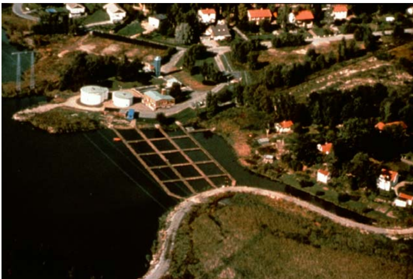
Figure 19. FBM installation located at Lake Trehormingen, Sweden (Karl Dunkers, Inc.).
